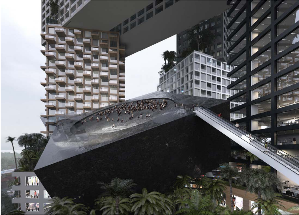
[Figure 5] MVRDV's Peruri 88 sky park view.
